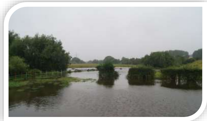
Figure 17: Flooding at Cotes Bridge, taken from the footpath on the A60
